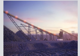
Mining Mobile stacking conveyor Barrick Gold
